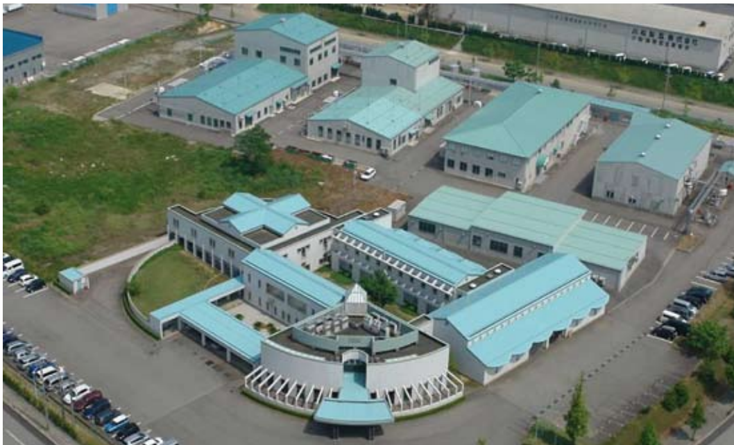
YMC Co., Ltd. manufacturing facility in Komatsu, Japan
